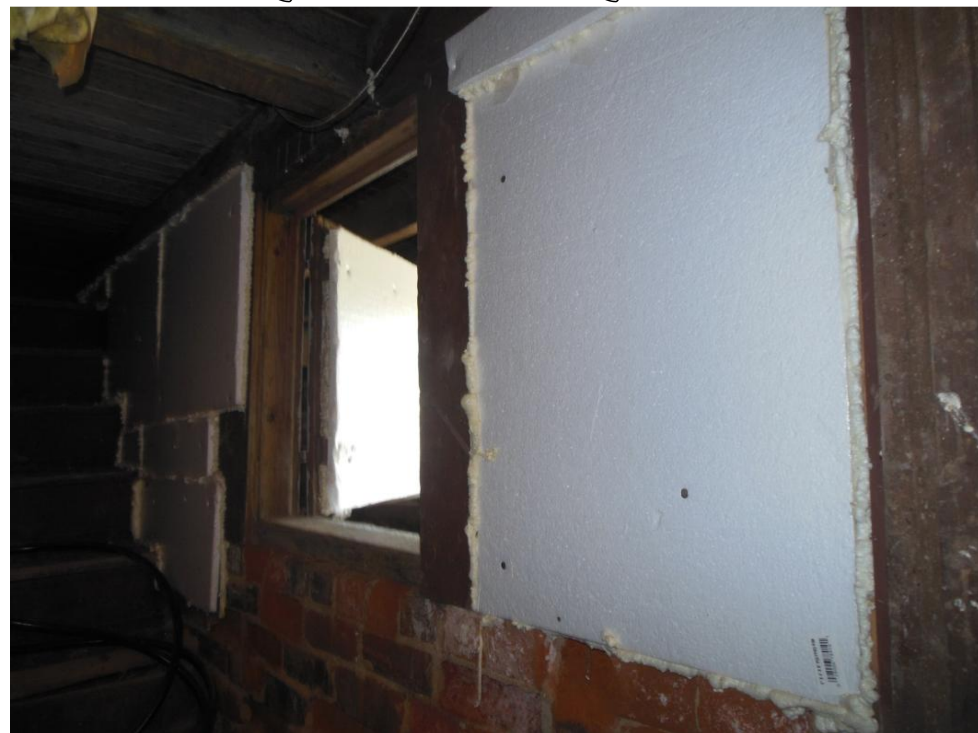
Rear Suite House Basement Access (Existing - 'Before')
