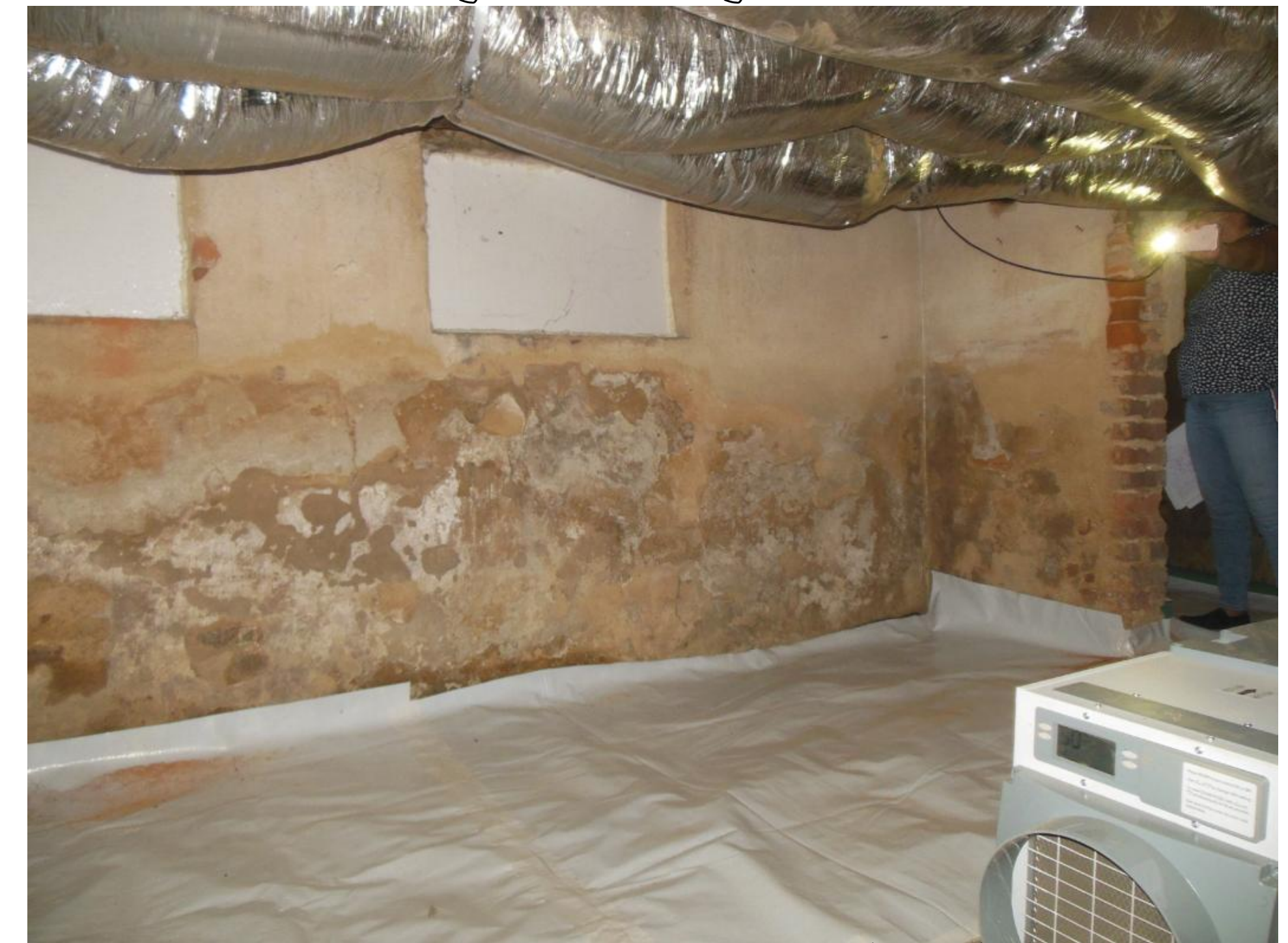
Rear Suite House Basement (Existing - 'Before')
