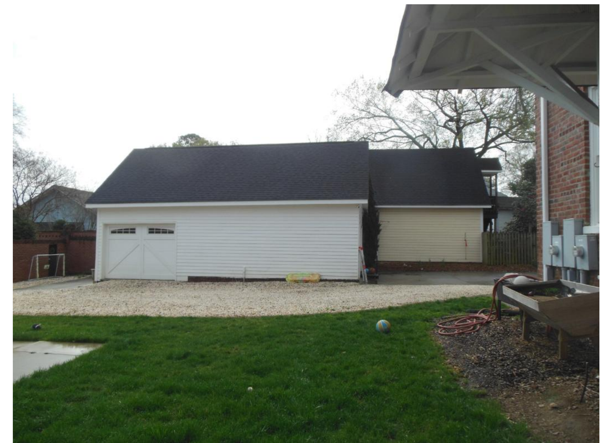
Left Side Garage Elevation (Existing - 'Before')
