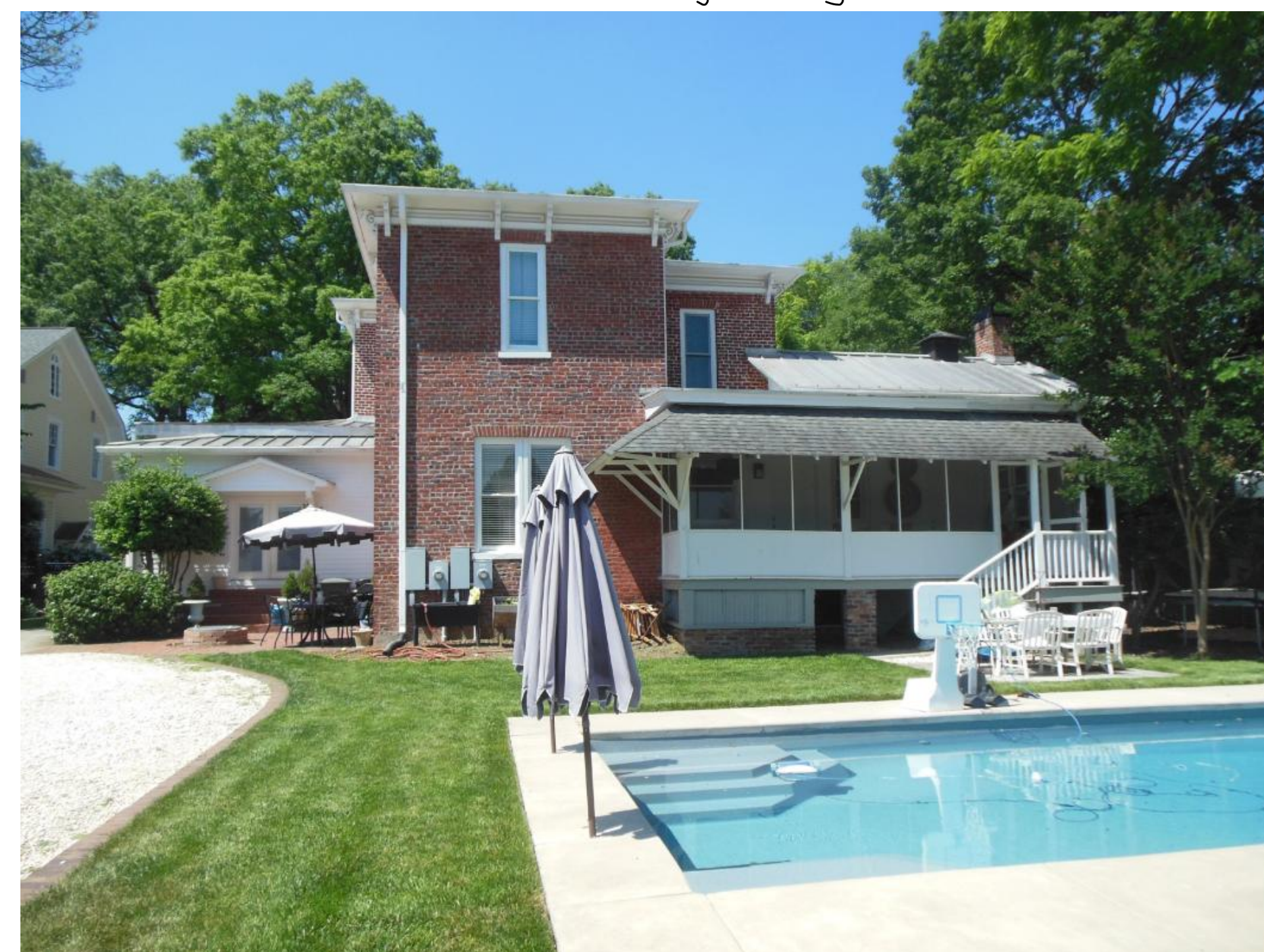
Rear House Elevation (Existing - 'Before')
