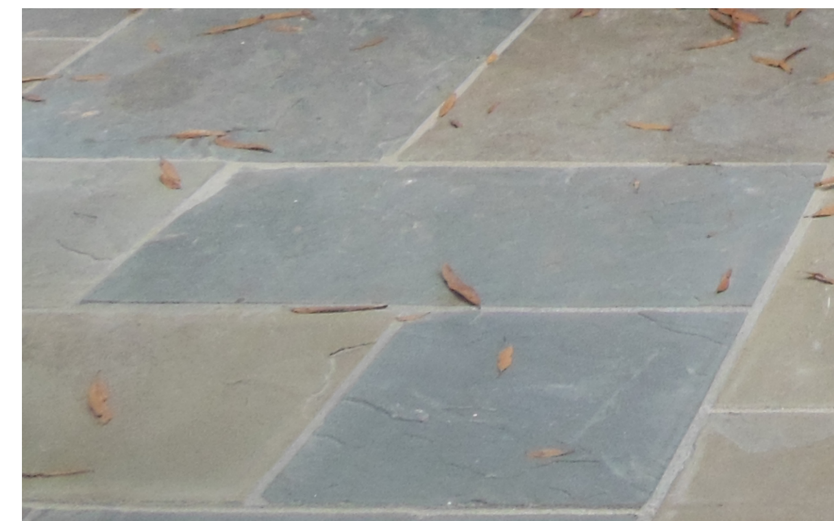
Bluestone Paver (Ashlar Pattern; New Covered Porch, Raised Terrace & Patio)
