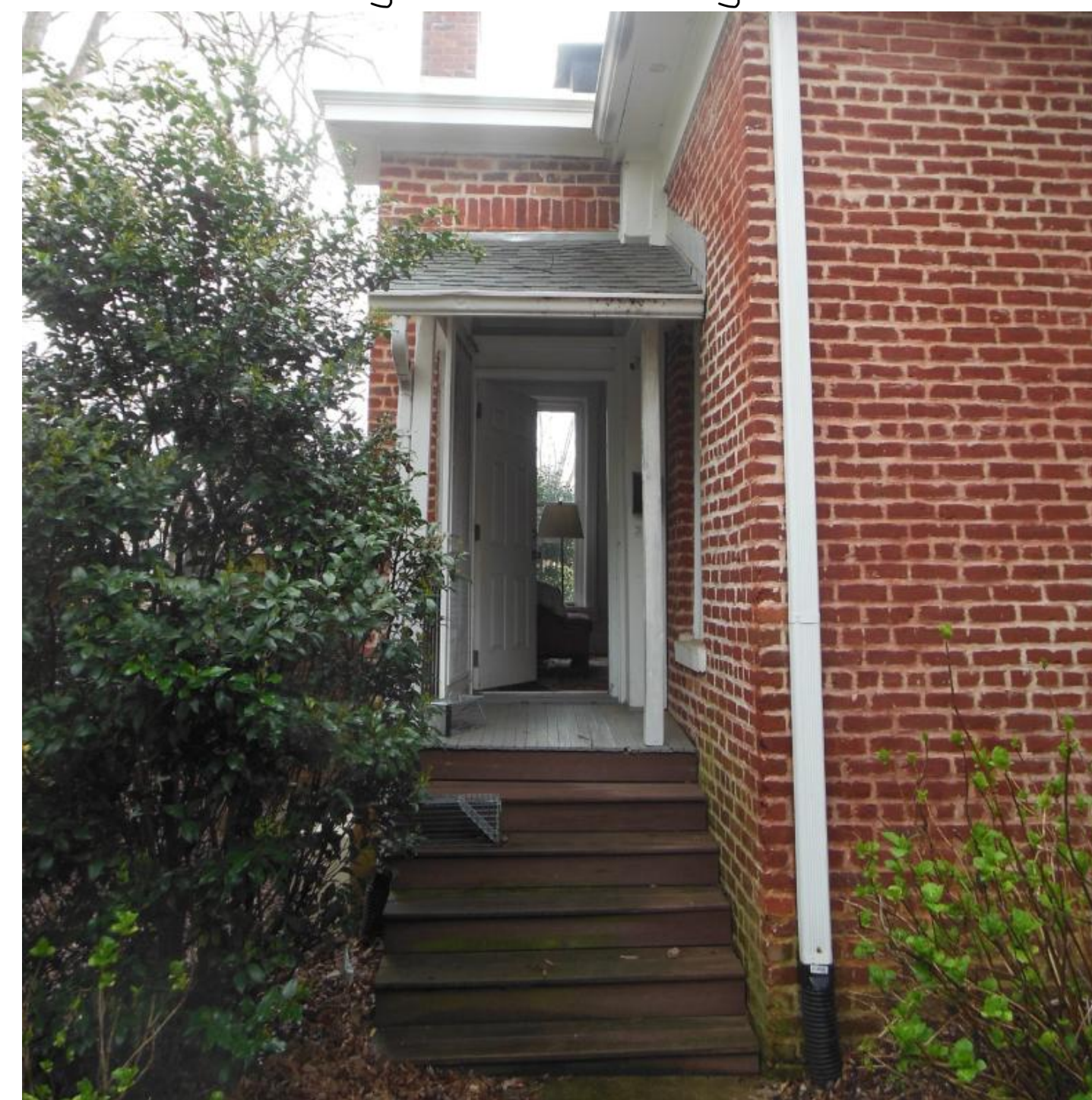
Front House Suite Side Entry (Existing - 'Before')
