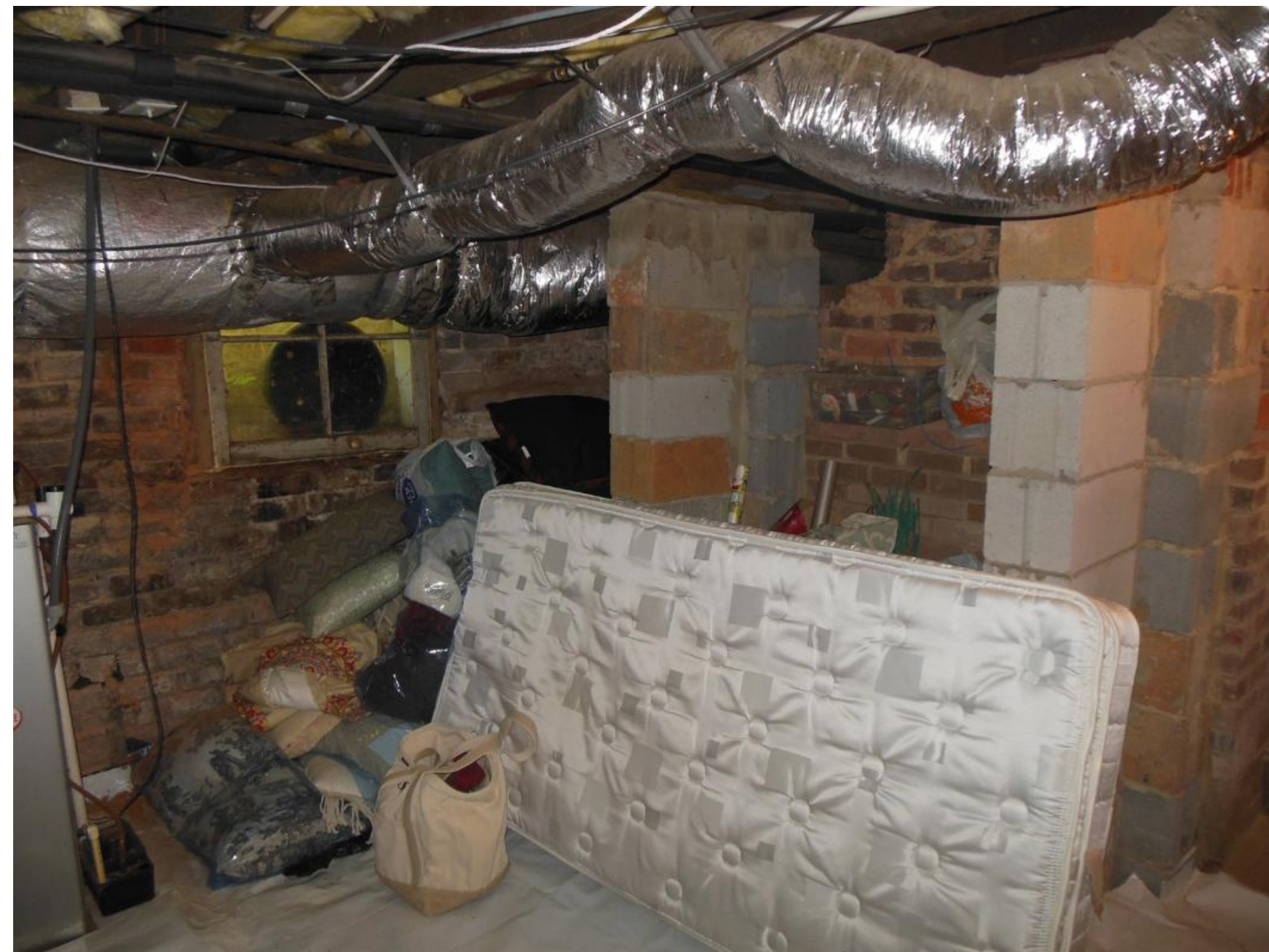
Original House Basement (Existing - 'Before')
