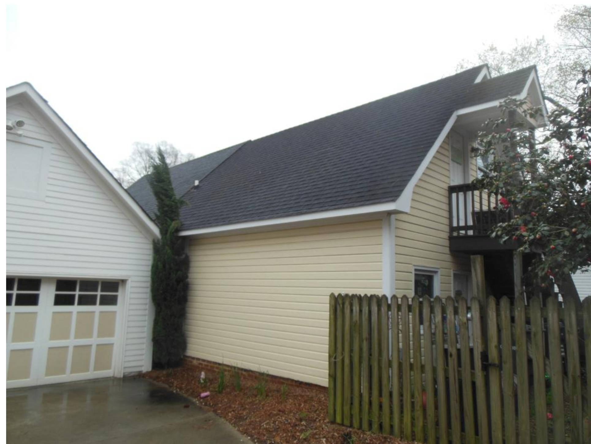
Neighboring Garage Structure (Existing - 'Before')
