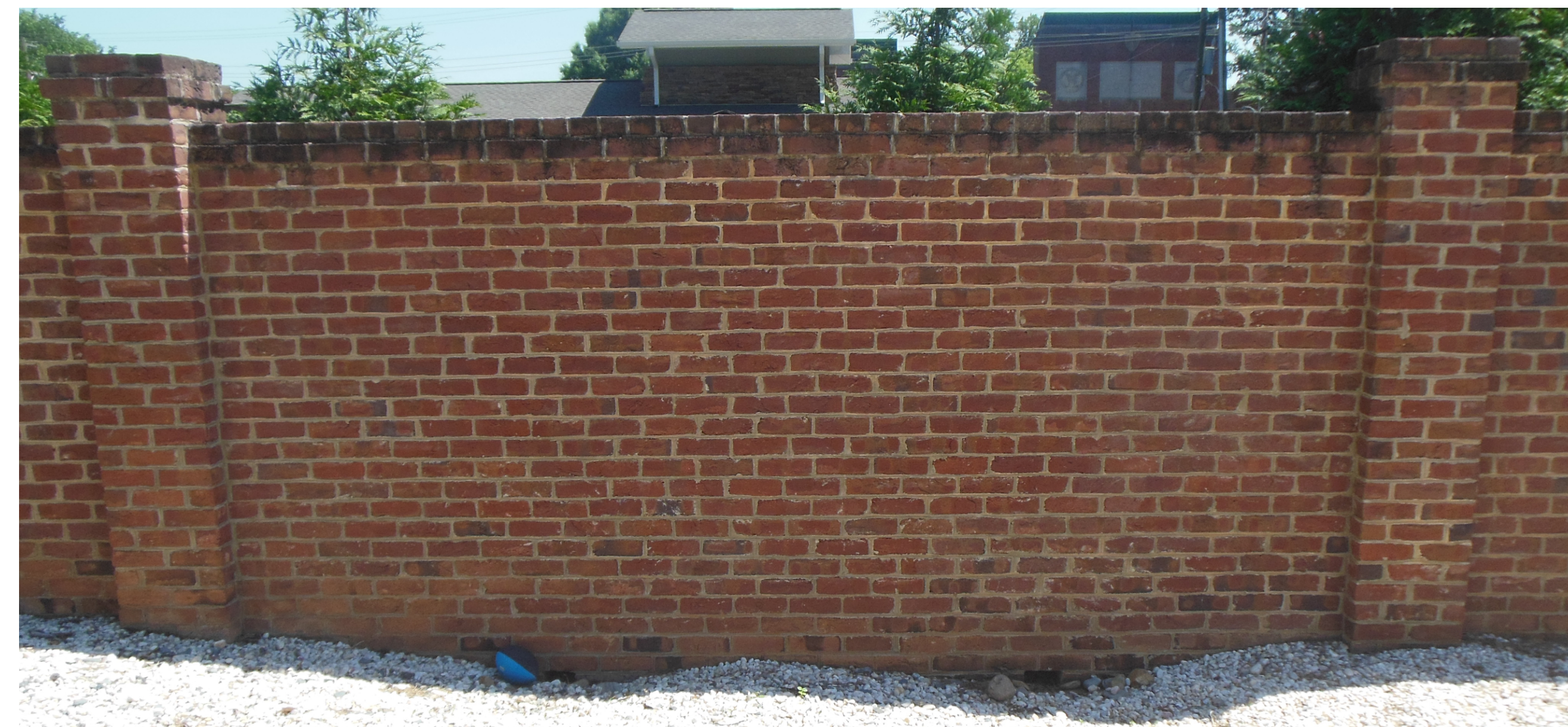
Brick Screen Wall (New Mechanical Areaway Screen Wall/Piers)
